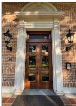
New museum front doors were installed in the fall.
